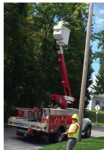
New Wilmington Borough lineworkers Chris Bowersox and Dean Ligo replace mercury vapor street lamps with LED lamps.
