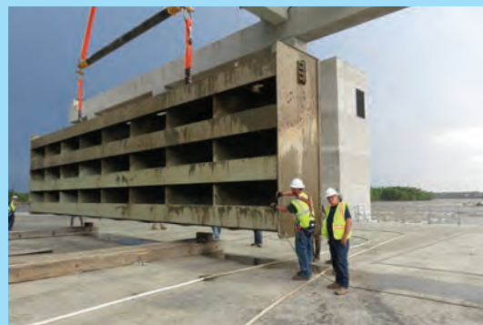
Mike Dabolt (right), AMP's Smithland O&M manager, oversees the last bulkhead being removed at the Smithland project.
