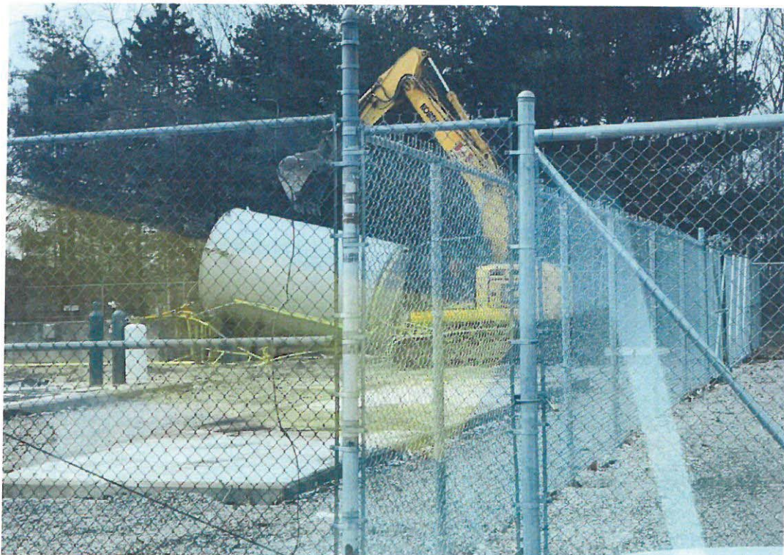
PHOTO 10: The AST being placed on the ground prior to cutting it up.
