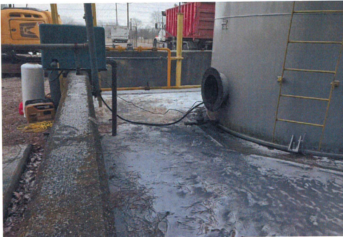
PHOTO 3: View of the inside of the AST dike. B&B Wrecking had to remove 200 gallons (4 drums) of fuel from the bottom of the AST before it could be demolished.
