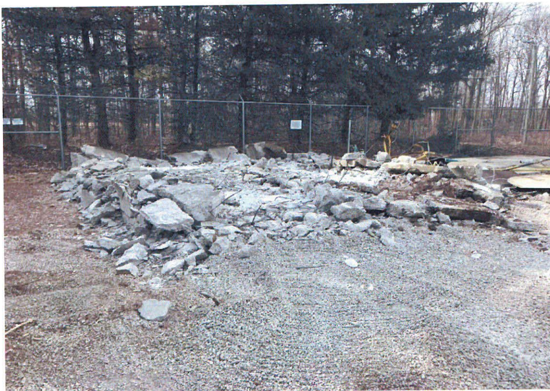
PHOTO 12: AST pad and dike. Concrete broken up with a hydraulic hammer mounted on a excavator.
