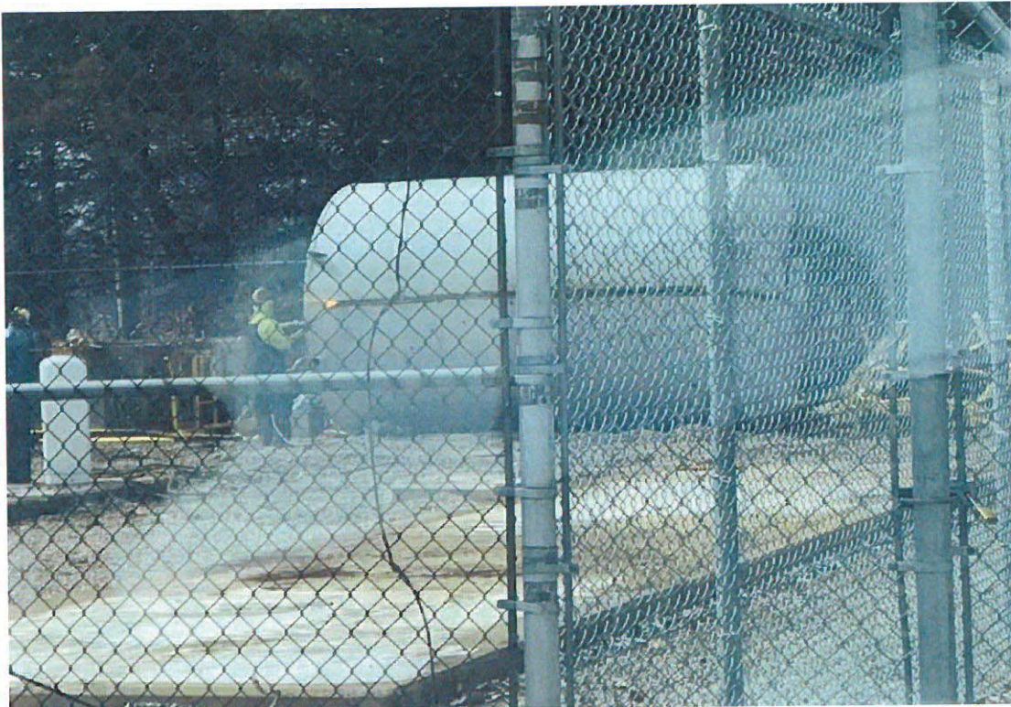
PHOTO 11: Cutting up the AST.
